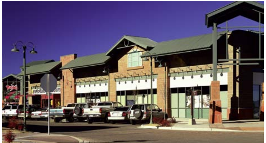
Liquid-applied fluoropolymer coatings have compiled a long and impressive track record of performance in demanding architectural applications, the result of the technology’s superior durability in exterior exposures. (Top): Metal panels at the Century Tel Center sports arena in Bossier City, LA, are finished with a beige-colored fluoropolymer coating. (Above): The rich color of the roof at the Prescott Gateway Mall, Prescott, AZ, was produced with a fluoropolymer coating. Photos by Wes Thompson.
