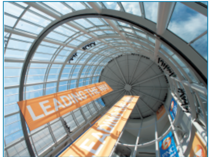
Solarban 60 glass by PPG transmits light into Prudential Center through two 110-foot-tall glass and steel cylinders.
