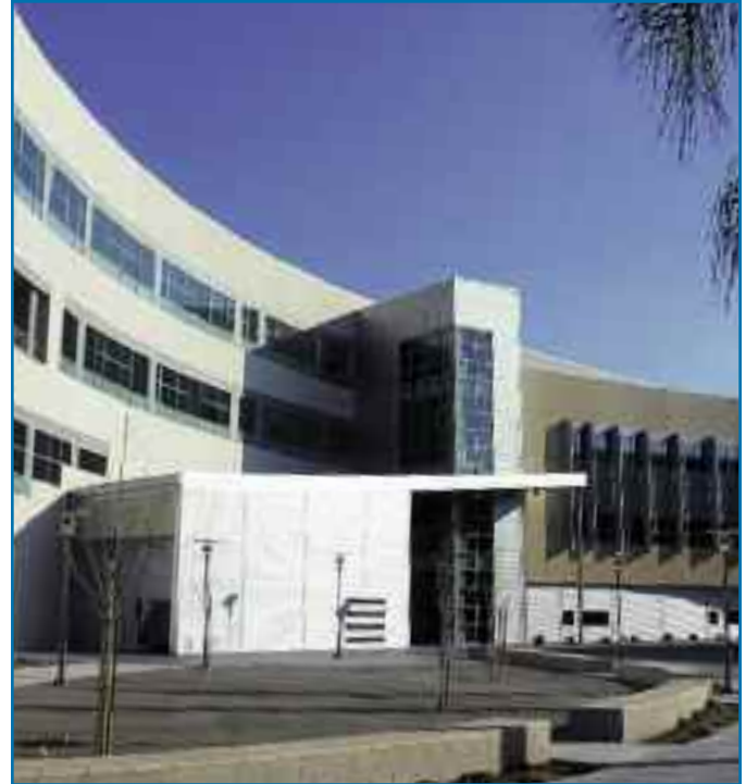
The College of Business Administration at California State University's San Marcos campus features Solarban 70XL glass, a revolutionary Solar Control Low-E coated glass that offers an unprecedented combination of visible light transmittance and solar control characteristics in a clear, color-neutral glass. Architect: A.C. Martin Partners, Los Angeles Glass Fabricator: Oldcastle BuildingEnvelope ™ Glazing Contractor: Division 8, Inc. CSUSM photo by George Cagala
