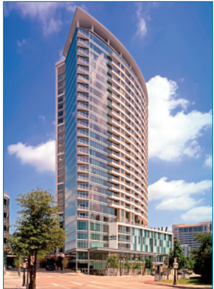
Cirque, a shimmering 28-story luxury apartment tower in Dallas, was designed with Solarban 70XL glass because of its excellent solar control performance and transparency.
