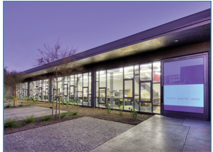
Architects HGW transformed a former gas station and auto repair shop into California's first net-zero-energy building with the help of Solarban 70XL glass by PPG.
