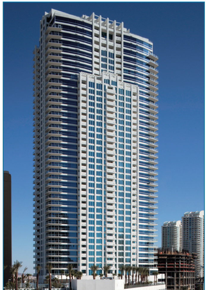
Sky Las Vegas, a luxury high-rise on the Las Vegas Strip, combines Vistacool Azuria glass and blue-tinted glass over Solarban 60 glass to maximize views and energy efficiency.
