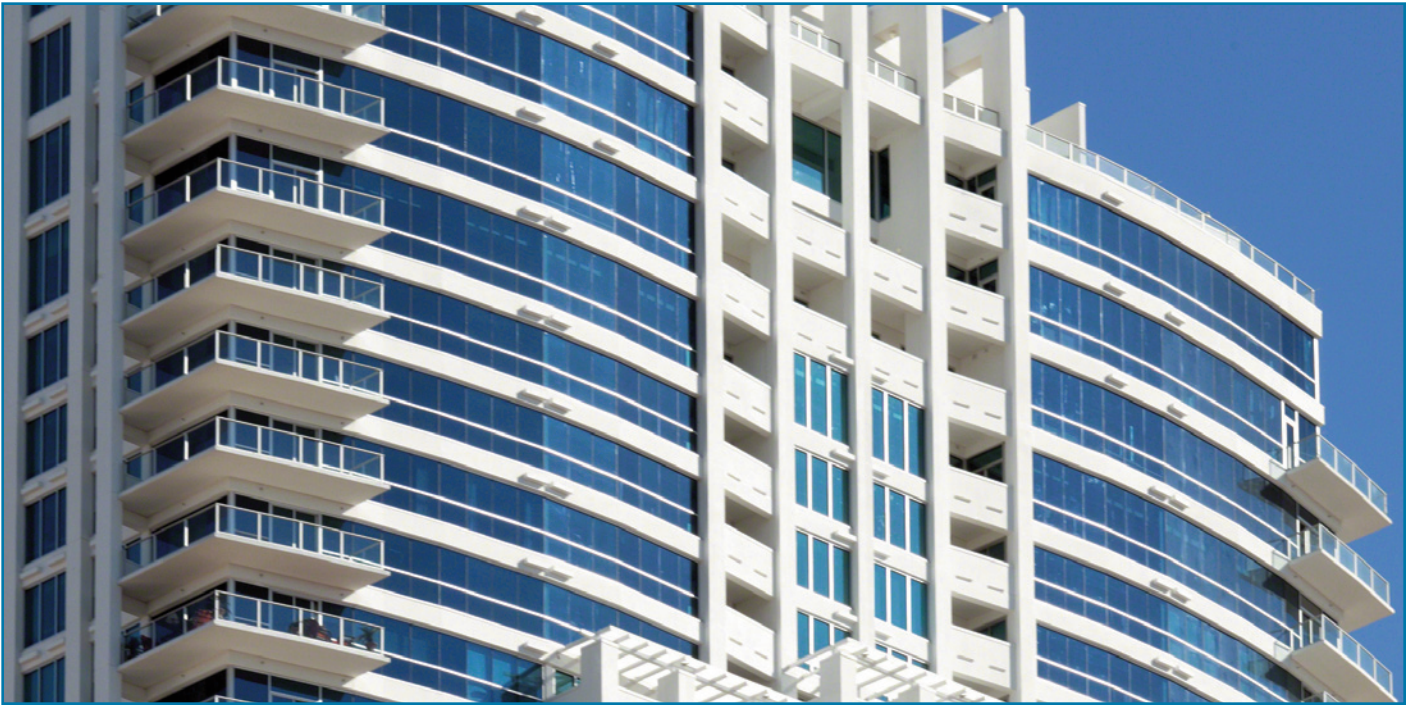
High-performance glazings by PPG control solar heat gain to help lower air-conditioning costs for residents of Sky Las Vegas.
